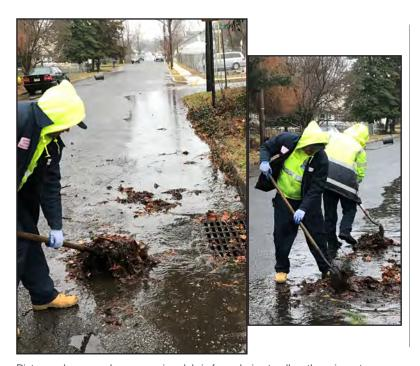
Pictures above: workers removing debris from drains to allow the rain water move down the sewer. Photos taken in the Blackwood section of Gloucester Township.
